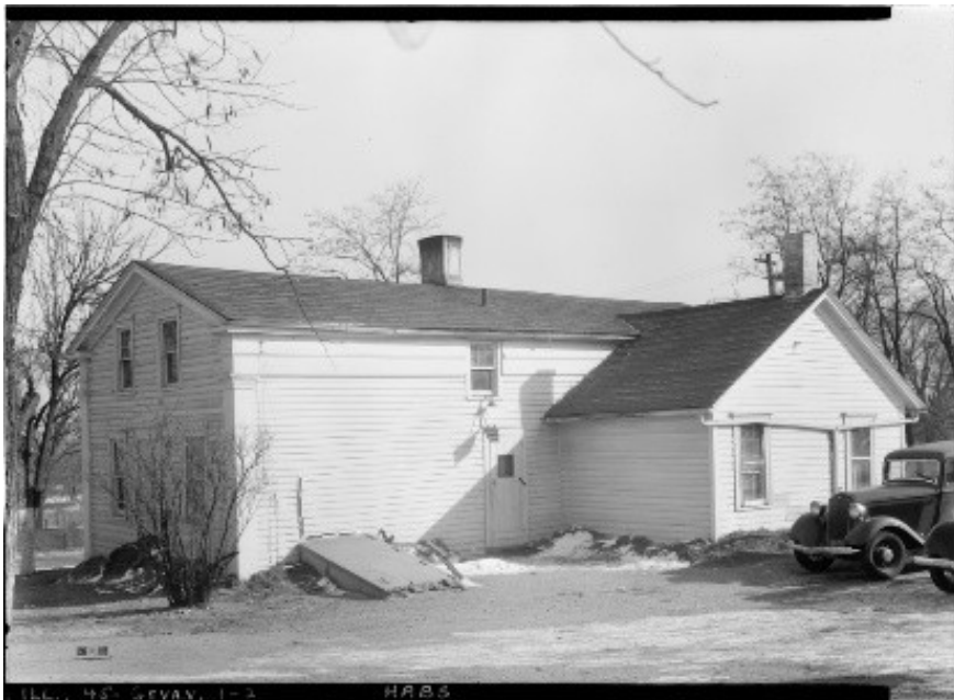
The back façade of the Bristol Farmhouse. The small sign over the rear door says "Entrance Bar Room." Notice that the north and south gable façades are the same with centered doors suggesting that the building is two small homes rotated and combined. (HABS, 1934)
